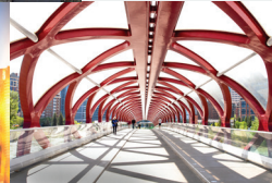
PEACE BRIDGE BY SANTIAGO CALATRAVA
